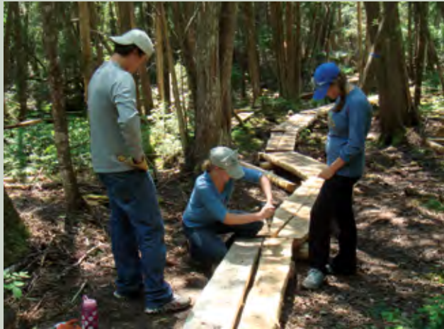
Volunteer trail crews installed hundreds of feet of cedar bog bridging through the wet areas, cleared brush and blow-down trees and marked the trails with small blue paint blazes.
